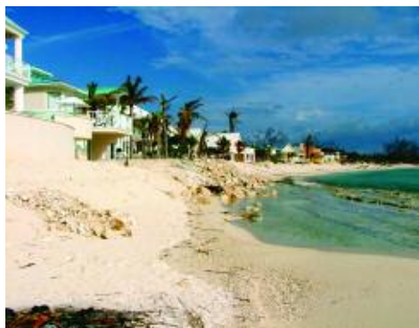
Coastal erosion in Cayman Island Credit: Department of the Environment, Cayman Island Government
