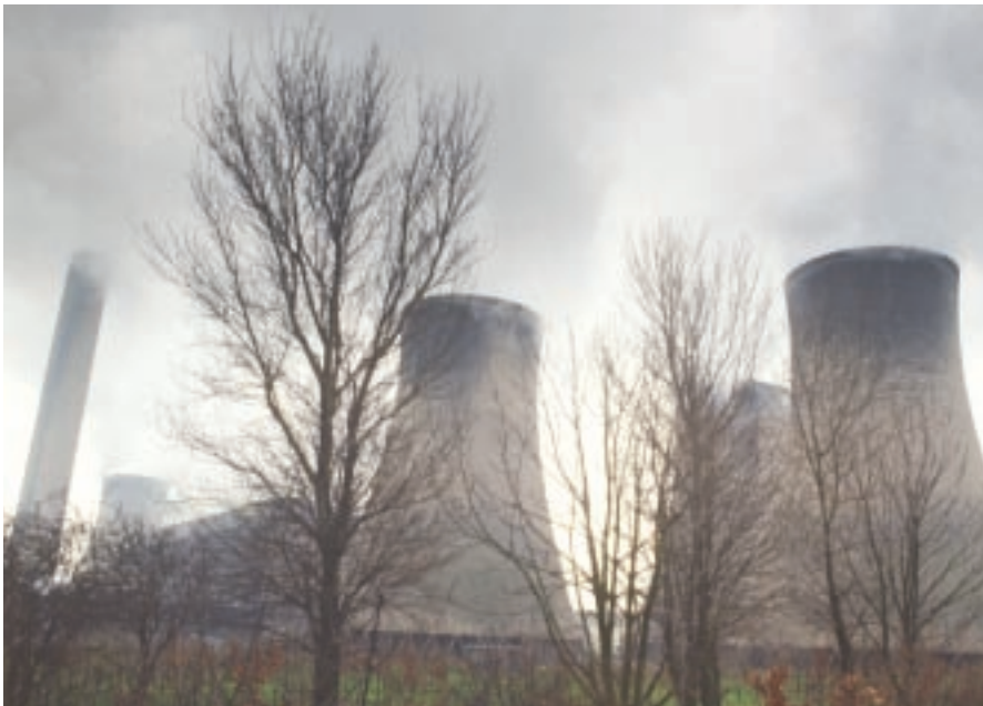
Fiddlers Ferry Power Station © Peter Wakely/English Nature
