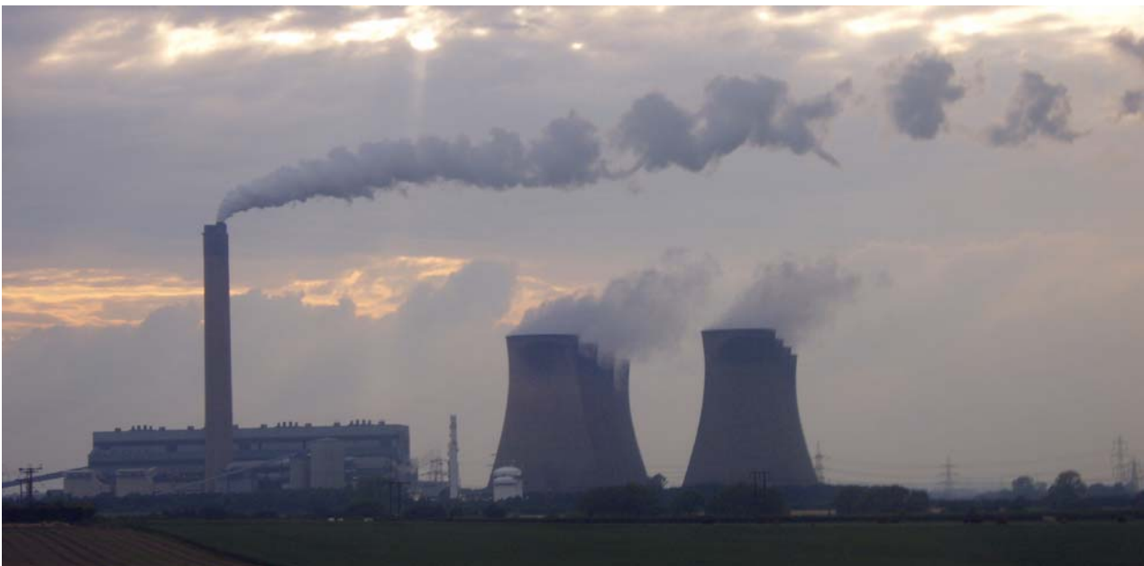
Power Station. Photograph by Cathy Gardener, JNCC 2007.
