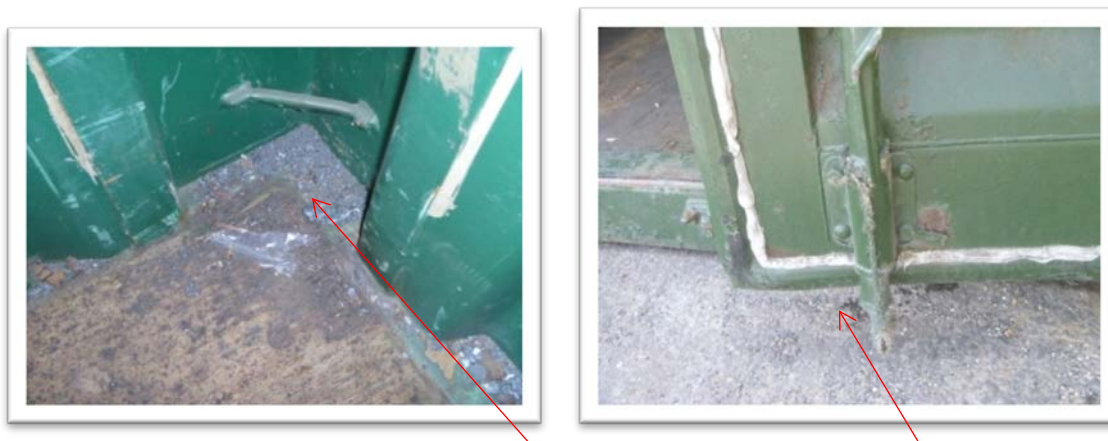
Figure 1. Accumulation of detritus, location of millipede and very old door seals
