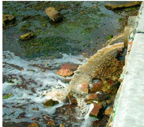
Wastepipe flowing into Stanley Harbour,
